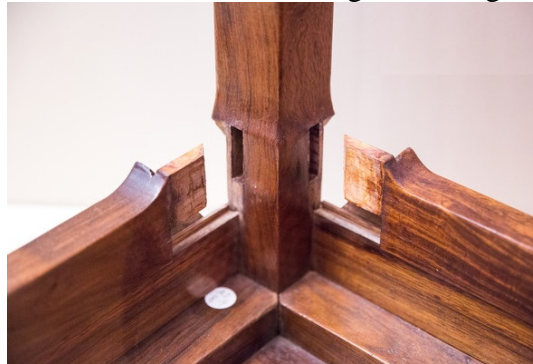
Figure 2: Mortise and tenon joint structure
